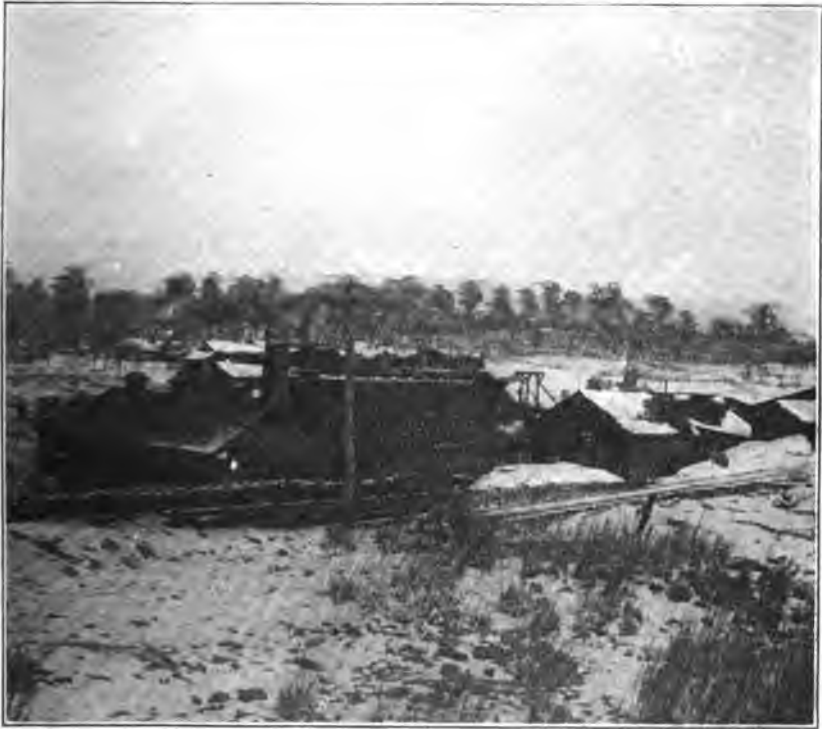
CHEMICAL REDUCTION PLANT HAILE GOLD MINE.
